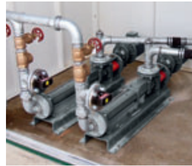
Waste water pumping
