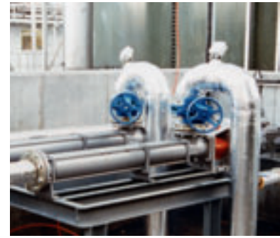
Pumping of slurry mix
