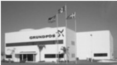
GMX - Monterrey, Mexico
