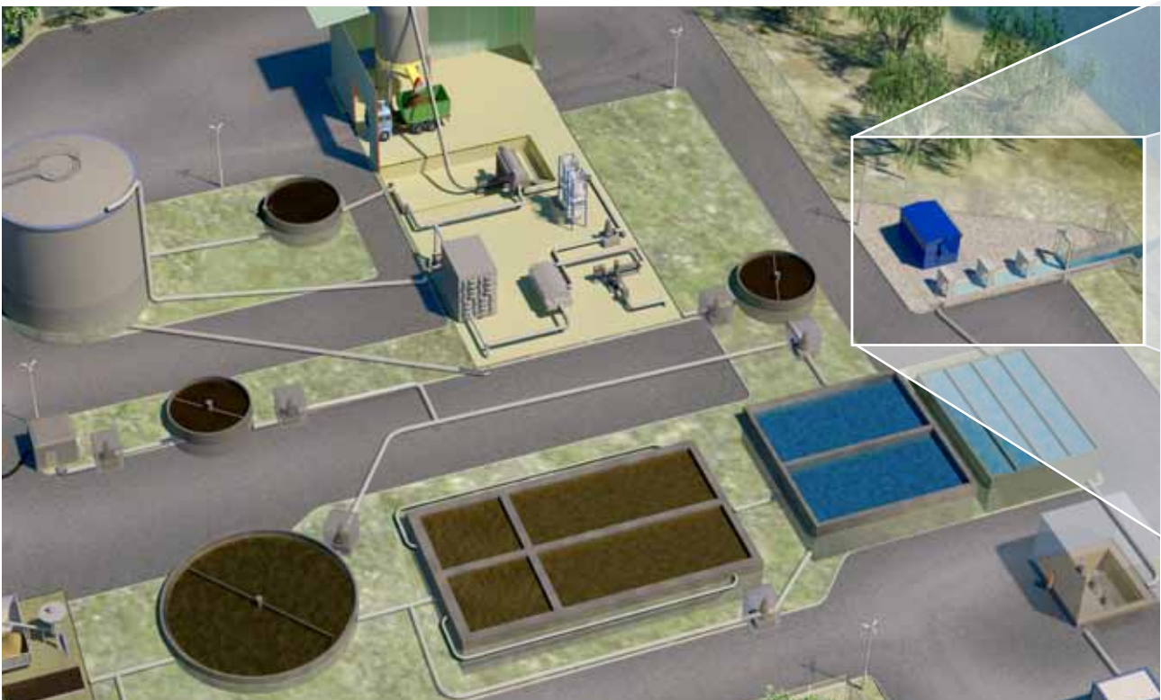
Overview of a typical waste water treatment plant with WEDECO TAK 55 UV disinfection as final treatment stage
